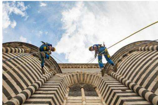
**Acrobatica** carries out external renovation works using **double safety rope** techniques.
